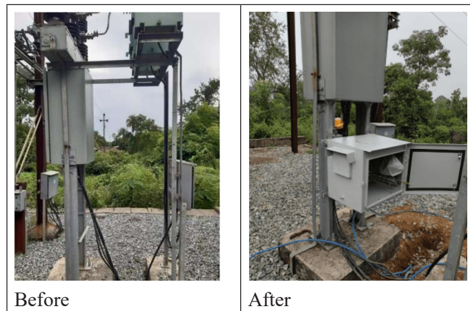
Fig. 3. Installation of micro-CRP
