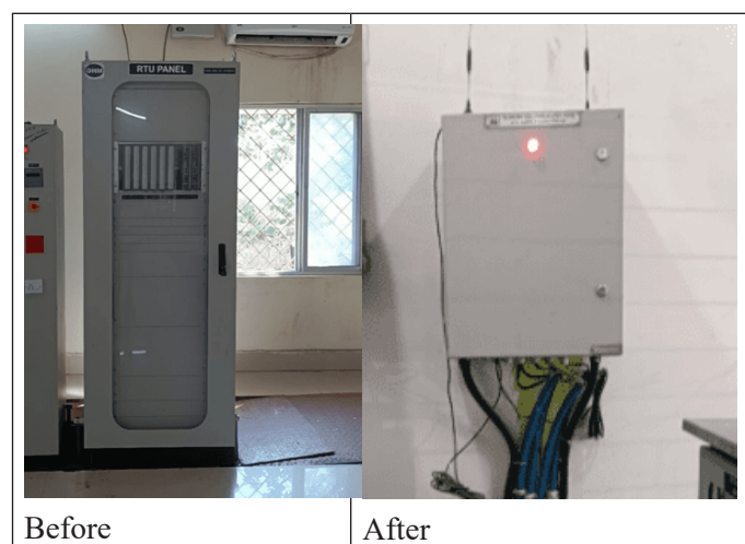
Fig. 4. Installation of RTU
